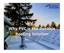
water-resistant polymer reinforced with fibreglass non-woven mats or polyester woven scrims. These roofing components ensure PVC's dimensional stability, durability, and capacity to respond to a building's normal expansion and contraction and resiliency challenges.
