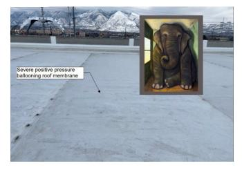
During the winter, warm-conditioned air entering under the roof membrane could lead to moisture condensation issues. The proposed solution includes sealing gaps, cracks, and openings, followed by roof restoration. The extent of "crackage" is estimated using satellite imagery, performed by on-site assessments of building envelope solution experts for precise documentation and pricing.
