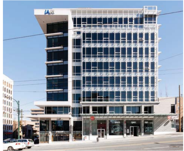
View Smart windows in a Broadway office tower darken in reaction to sunlight or with the use of a mobile app • SUBMITTED
